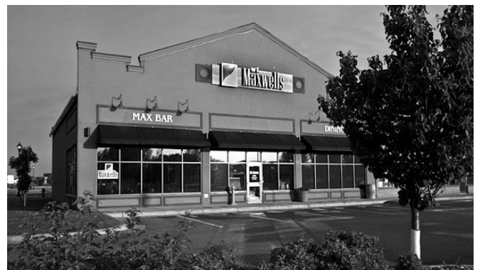
(Mall at 13th Avenue & 9th Street E., West Fargo)
